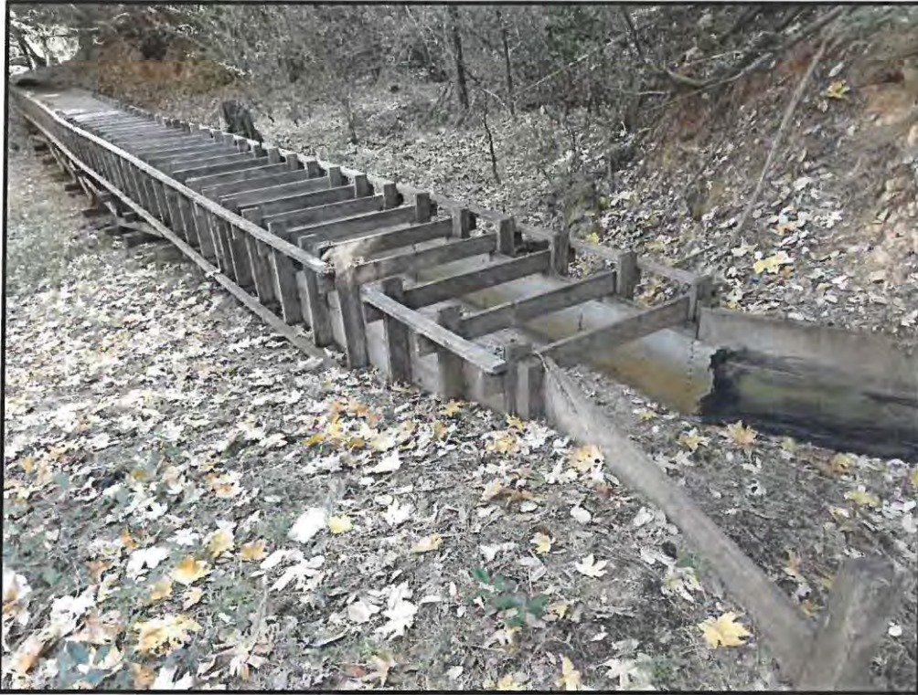
PHOTO - 7 A wooden flumed section of the ditch.
