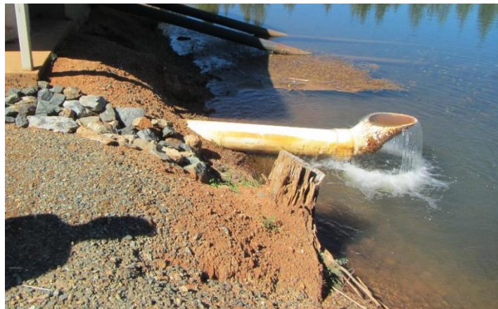
Photo 0624: Water from ditch emptying into NYWD reservoir; possible RSW-001 location. Photograph taken by State Water Board staff Jacques Lord, on July 11, 2019.
