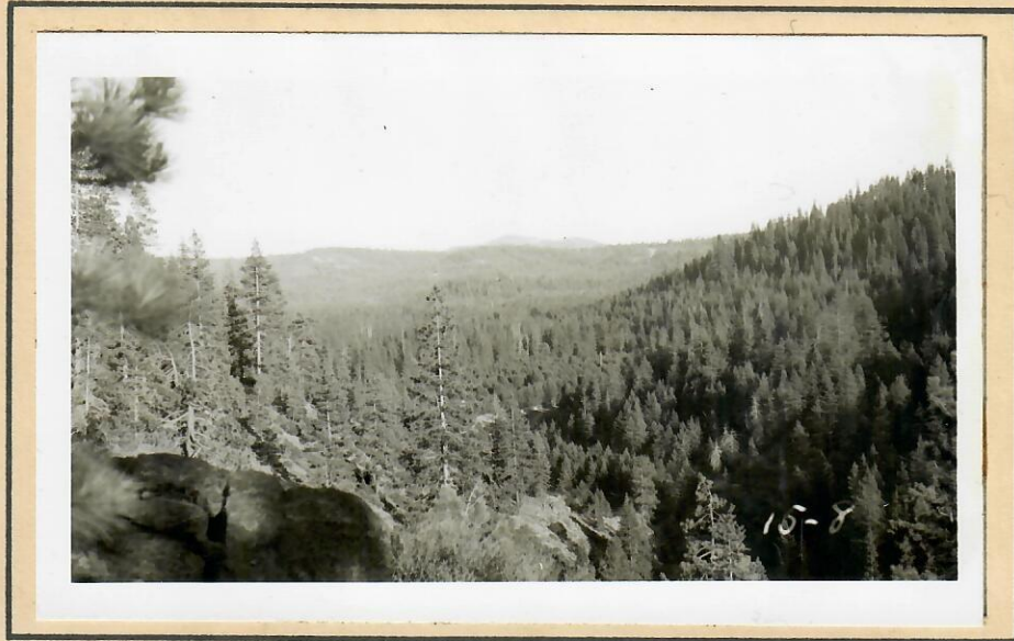
LITTLE GRASS VALLEY DAMSITE
