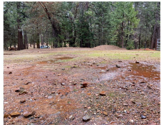
Robert Summa/Appeal-Democrat Water collects near a leak of the tank that supplies water to customers in Forbestown on March 14.
