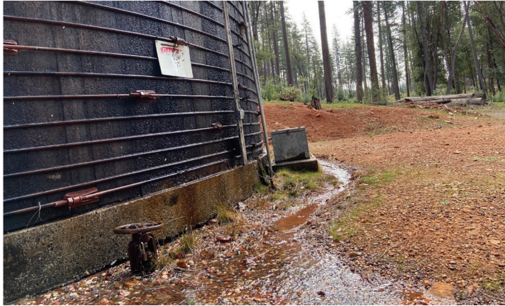
Robert Summa/Appeal-Democrat Water is pictured streaming from the leak of a water tank that supplies treated water to North Yuba Water District customers in Challenge.
