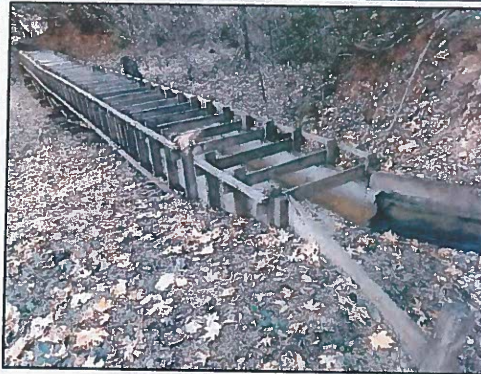
PHOTO - 7 A wooden flumed section of the ditch. -Standing on the southern side of the ditch/flume looking northeast. 5 NOV 2019
